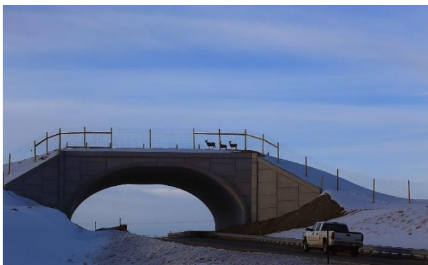
Highway 9 Wildlife Crossing (Photo from CPW)
